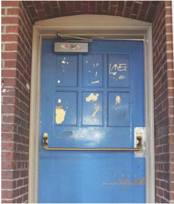
2.5.3/4 Painted-over door lights at Building C mezzanine. Also note historic hardware.
