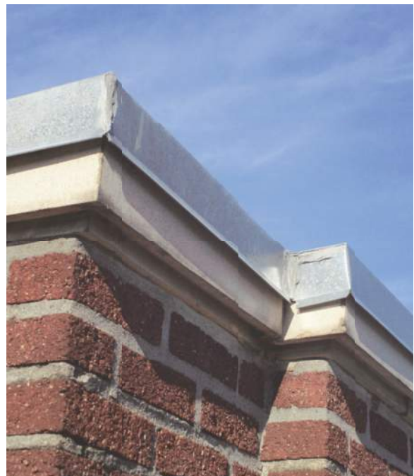
2.2.4/14: Galvanized sheet metal flashing installed at parapet coping, Building A - east elevation. Note open seams at corners covered with sealant.
