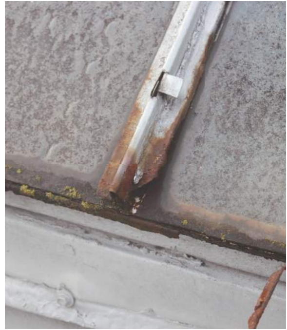
2.4.3/2 Skylight E11: Typical existing biogrowth, corroded metal components and deteriorated sealant on historic skylights.
