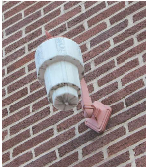
2.7.1/8 Fixture H: exterior metal sconce.
