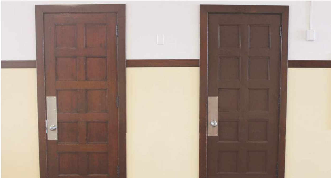
2.5.2/1 Two doors at the second-level lobby of Building B. The left one is wood and the right door is clad with sheet metal.
