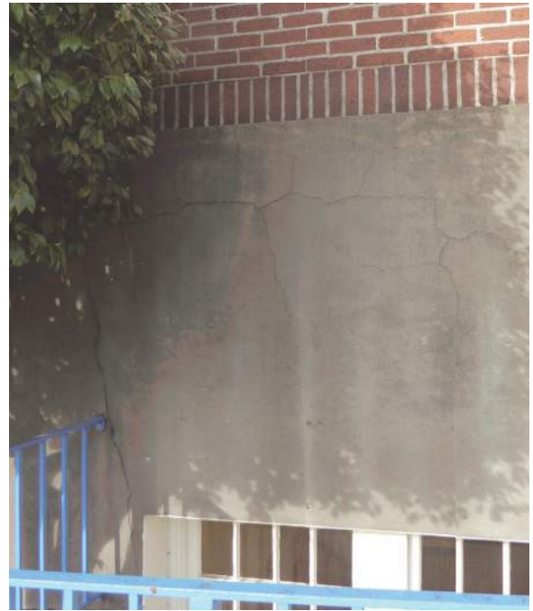
2.2.3/18 Superficial parge coat cracks.
