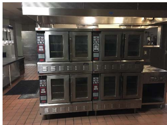
Existing Convection Ovens
