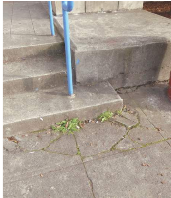
2.2.3/14 Cracks and biogrowth seen at walkway pavers.
