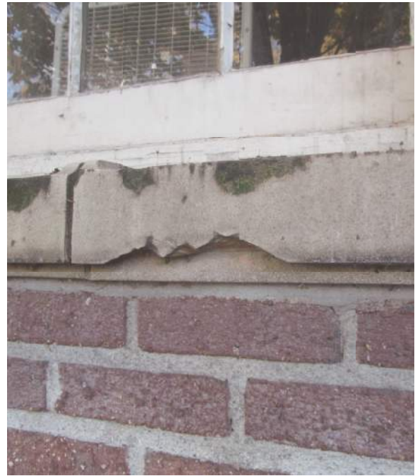
2.2.3/32: Large losses at terra cotta window sills, Building G - north elevation. Also note soiling and biological growth. Spall damage most likely related to vandalism.
