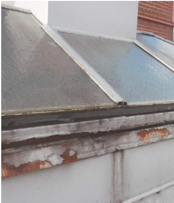
2.4.3/3 Skylight E13: Typical corroded metal flashing, biogrowth, and peeling paint on historic skylights.
