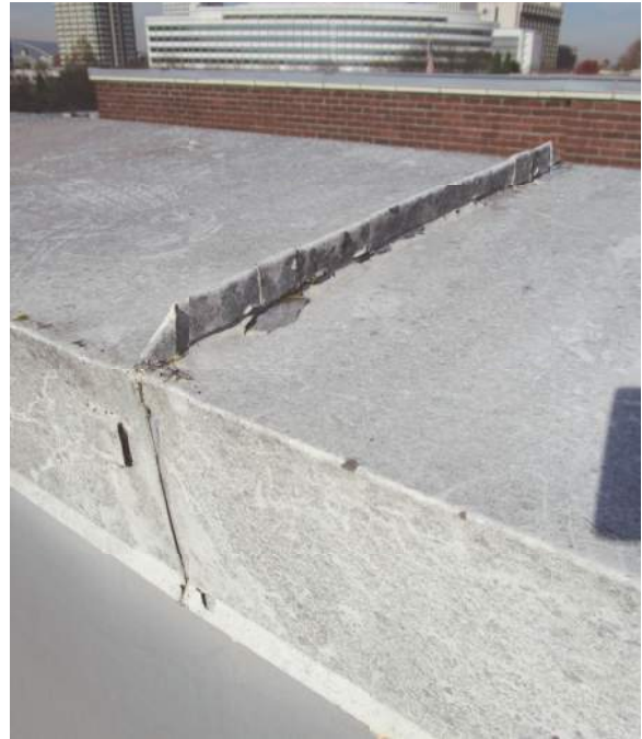
2.2.4/12: Damaged seams and peeling paint at galvanized sheet metal flashing, Building C - north elevation.
