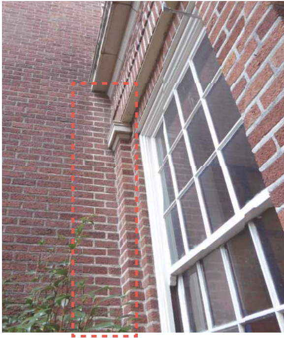
2.2.2/1 Area of protected masonry that shows clean mortar joints.
