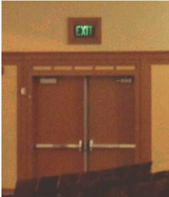
2.7.1/5 Fixture E: illuminated exit sign.
