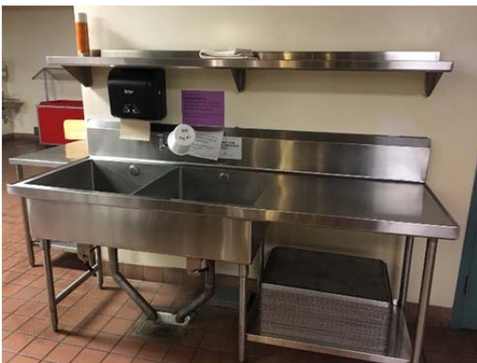
Existing Prep Sink
