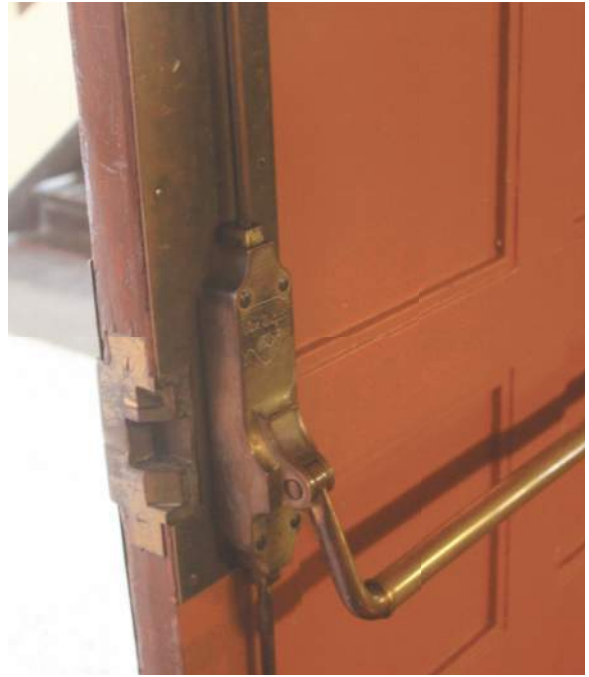
2.5.3/5 Historic pushbar hardware at Building B cafeteria doors.
