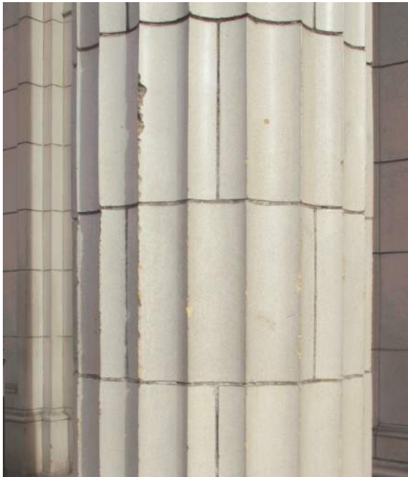
2.2.3/31: Chip losses and abraded edges at fluted column units, Building A - west elevation portico.
