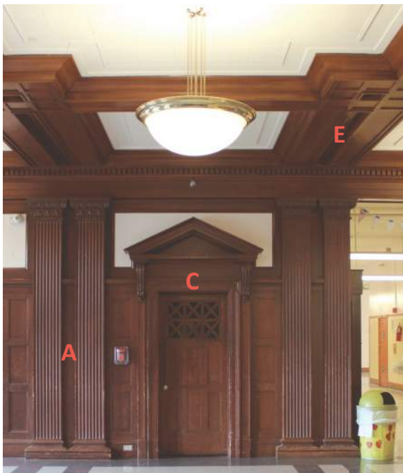
2.6.1/1 Interior door with wood pediment flanked by paired stained wood Doric pilasters and paneled wainscot.
