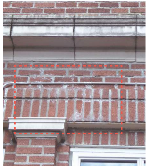
2.2.3/10 Area showing heavy efflorescence at mortar joints.
