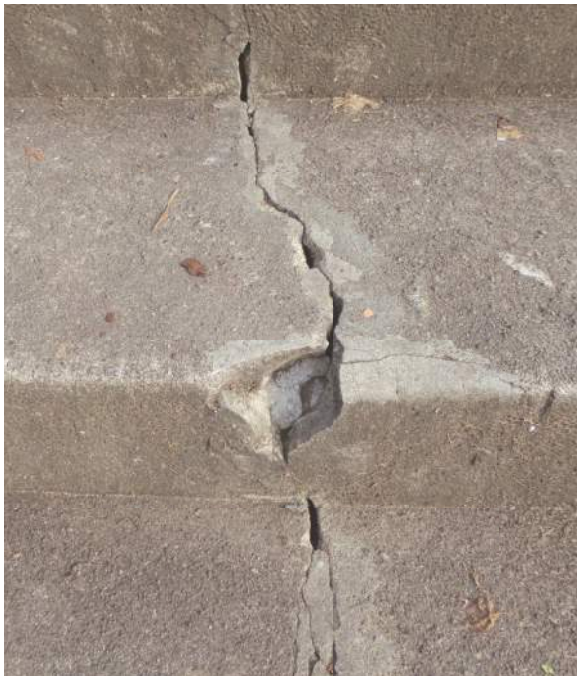
2.2.3/15 Failed concrete patch at exterior stairs.
