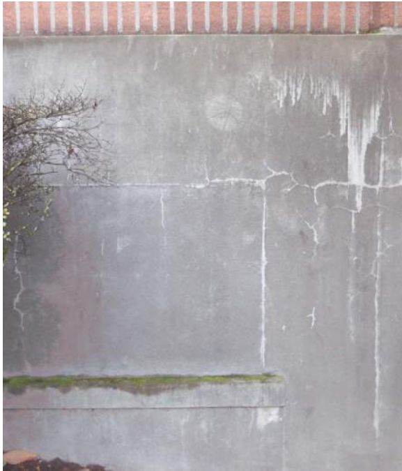
2.2.3/21 Crack in parge coat following outline of window infill.
