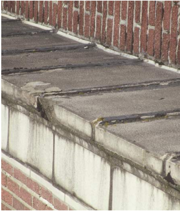
2.2.4/7: Deteriorated roofing mastic applied over upward-facing joints at terra cotta copings, Building A - south elevation.
