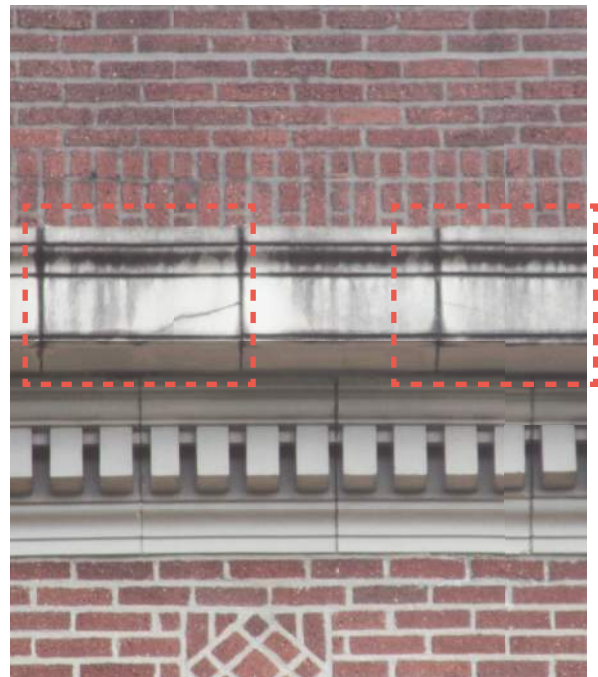
2.2.3/28: Two cracked cornice units at Building A - west elevation.
