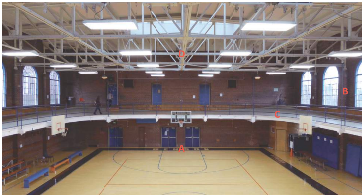
2.6.3/1 Old Gymnasium from mezzanine level.
