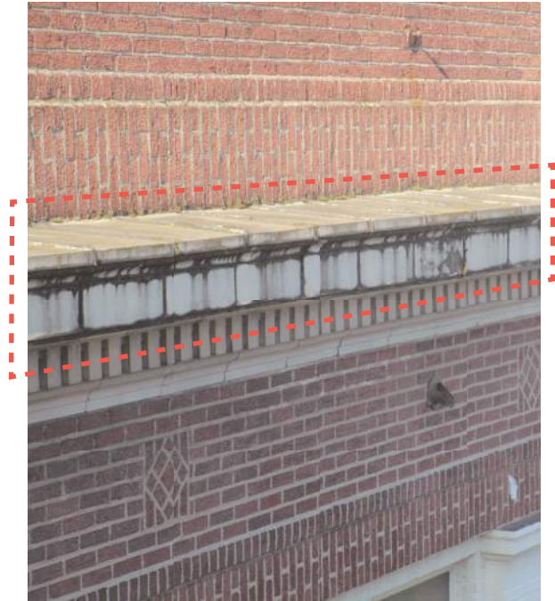
2.2.3/22: Heavy soiling, stains and biological growth at terra cotta cornice, Building C - north elevation.
