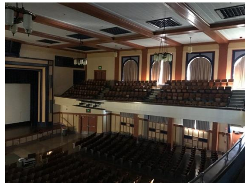
Balcony and Ceiling
