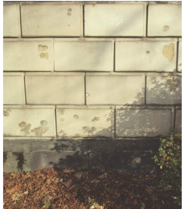
2.2.3/36: Glaze spalls at terra cotta stair wall, and cracking, water stains and efflorescence at concrete base, Building B - west elevation.
