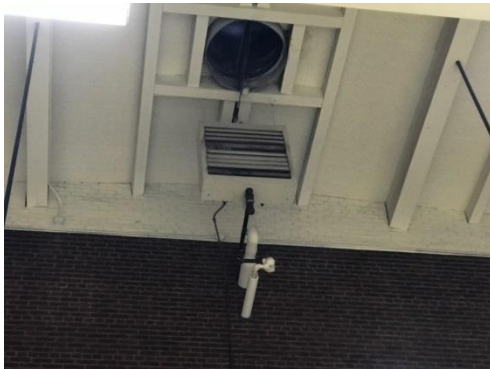
Noisy Mechanical Equipment
