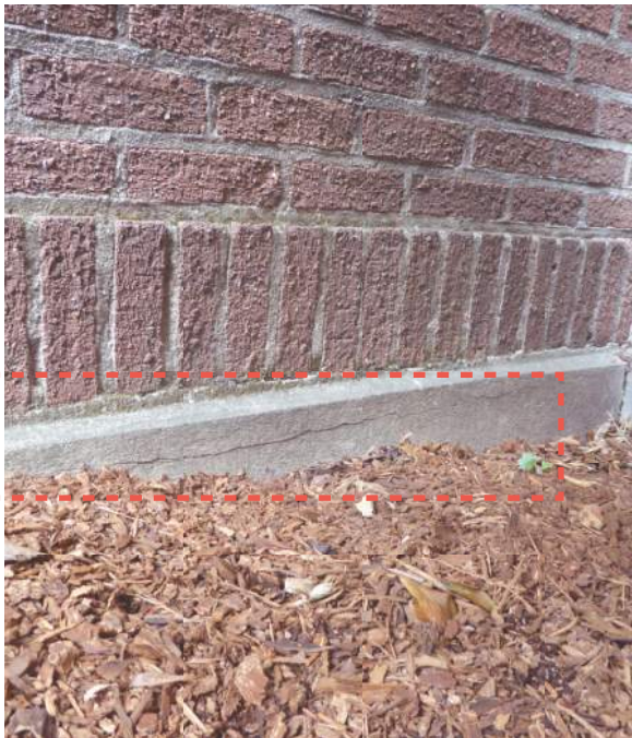
2.2.3/19 Crack in concrete sill.
