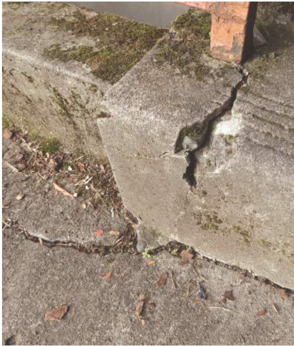
2.2.3/13 Concrete spalls and cracking.
