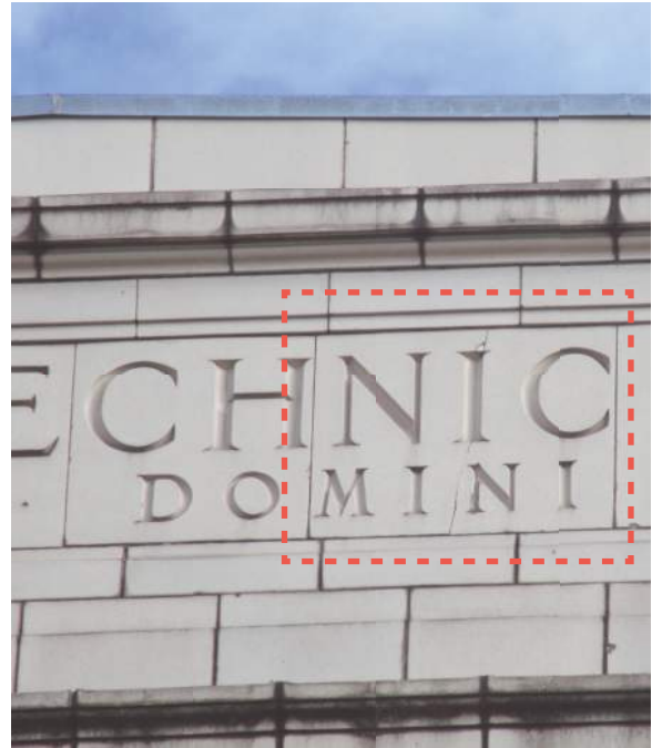
2.2.3/30: Two cracked cornice units at Building A - west elevation.
