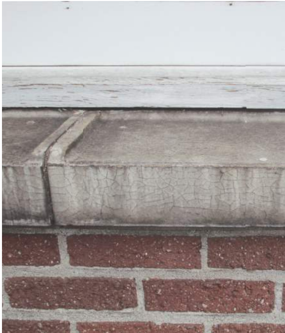
2.2.3/23: Crazing at first floor window sill units, Building A - west elevation.
