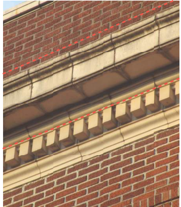
2.2.3/24: Eroded mortar and associated staining and glaze spalls at terra cotta cornice, Building C - north elevation.
