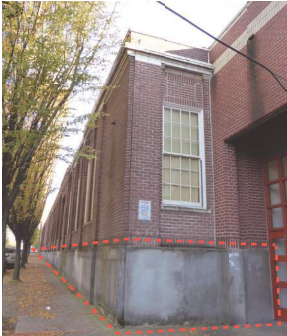
Photo 2.2.2/3 Above-grade foundation wall.
