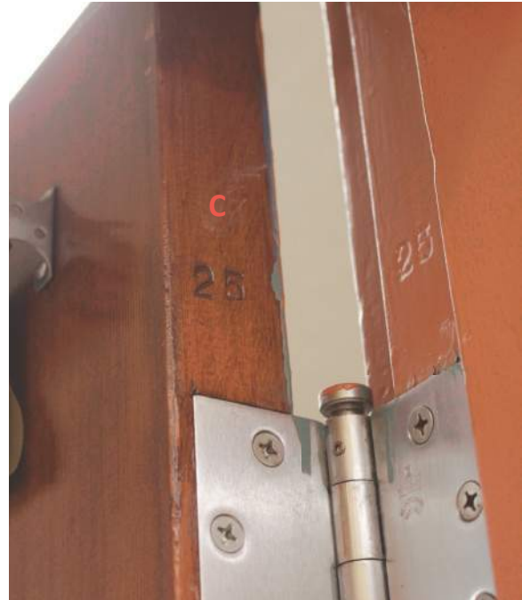
2.6.1/6 Original door number stamp on door and corresponding frame.
