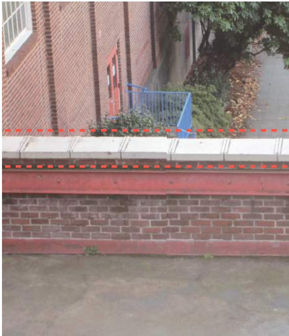
2.2.4/9: Section of original terra cotta coping at connection bridge between Buildings A & C. At most other locations, copings have been covered with sheet metal flashing.
