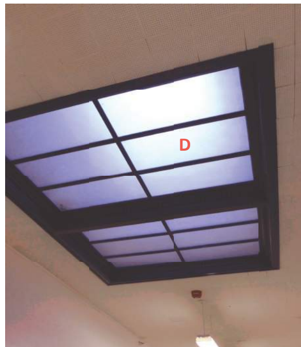
2.6.1/8 One of five multi-light skylights.
