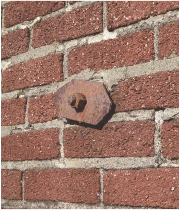
2.2.3/11 Steel wall tie at parapet of Building A.
