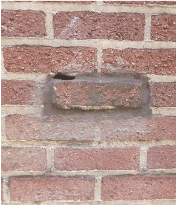
2.2.4/1 Brick unit needing to be removed and reinstalled with new mortar.
