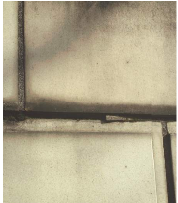
2.2.3/26: Detail of loose/spalling mortar at terra cotta stair wall, Building B - west elevation.
