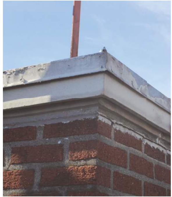
2.2.4/8: Painted sheet metal cap flashing installed over terra cotta copings at Building C. Note deteriorated coping joints and horizontal sealant joint between coping and brick parapet wall.
