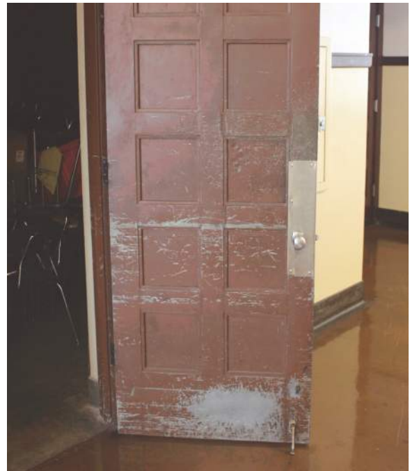
2.5.3/2 Dented and scratched kalamein door. Coating is severely abraded.
