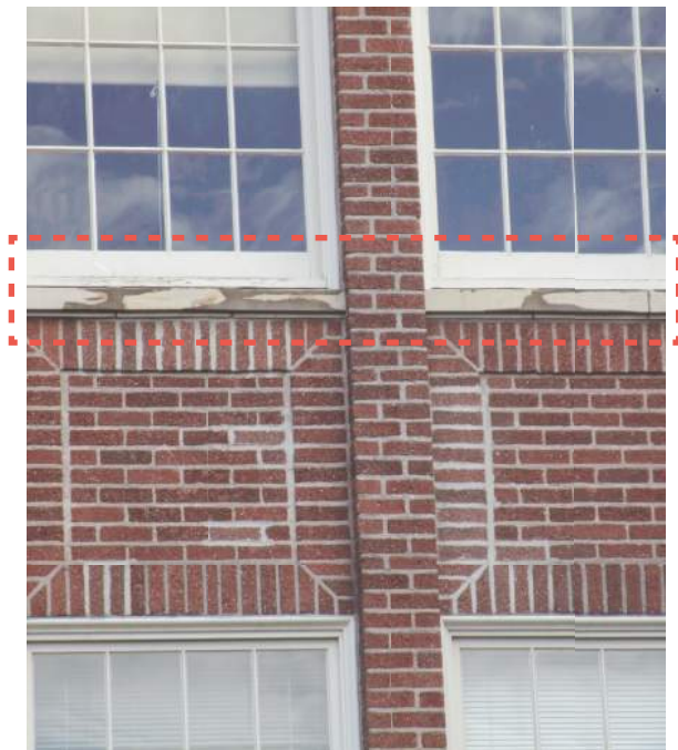
2.2.4/15: Previous cementitious patch repairs at terra cotta window sills, Building A - west elevation.
