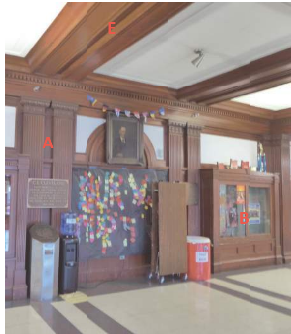
2.6.1/4 Wood display cases across from main entry doors. Also note box beams.
