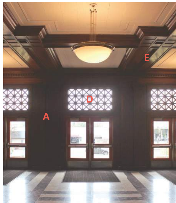
2.6.1/2 Multi-light transoms over main entry doors. Also note ceiling wood molding detailing.
