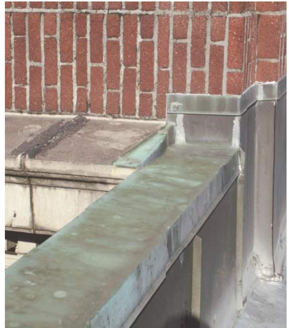
2.2.4/10: Copper sheet metal flashing installed at wall and parapet, Building A - east elevation.
