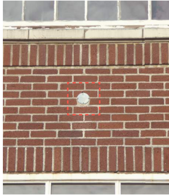
2.2.3/12 Escutcheon cover where light fixture was removed.
