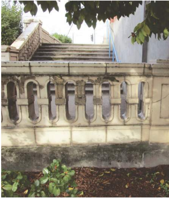
2.2.3/33: Cracking, glaze spalls, heavy soiling and biological growth at stair balustrade, Building B - south elevation.
