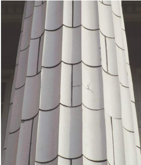
2.2.3/29: Cracks at fluted column unit, Building A - west elevation.
