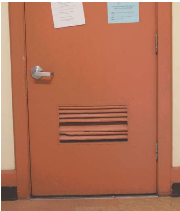
2.5.3/6 Typical broken slats at wood door grilles.
