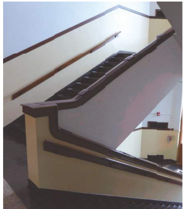
2.6.2/6 NW auditorium staircase from first floor.
