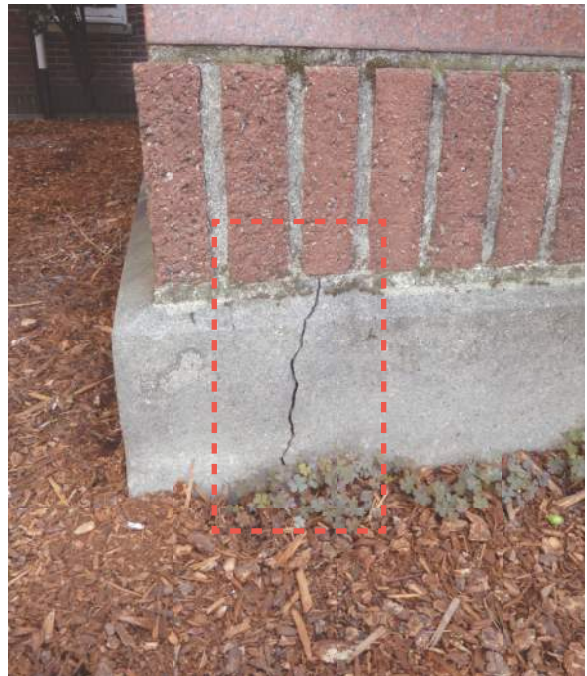
2.2.3/16 Structural crack in foundation at the NW corner of Building A.
