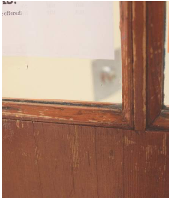
2.5.3/1 Typical door wood crack and split wood condition.
