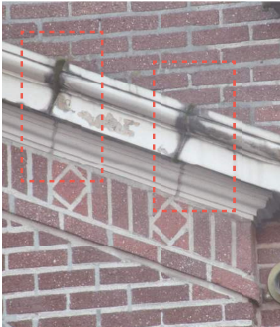
2.2.3/25: Detail of eroded mortar and associated staining and glaze spalls at terra cotta pediment, Building E - east elevation.
