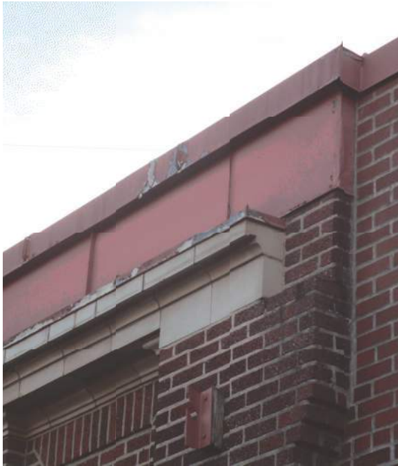
2.2.4/11: Painted galvanized sheet metal flashing covering entire parapet wall and coping; also cap flashing at cornice, Building J - north elevation. Note peeling paint throughout.
