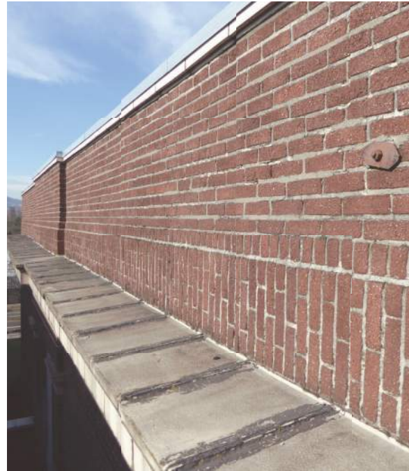
2.2.4/2 Mortar deterioration at parapet terra cotta unit joints.
