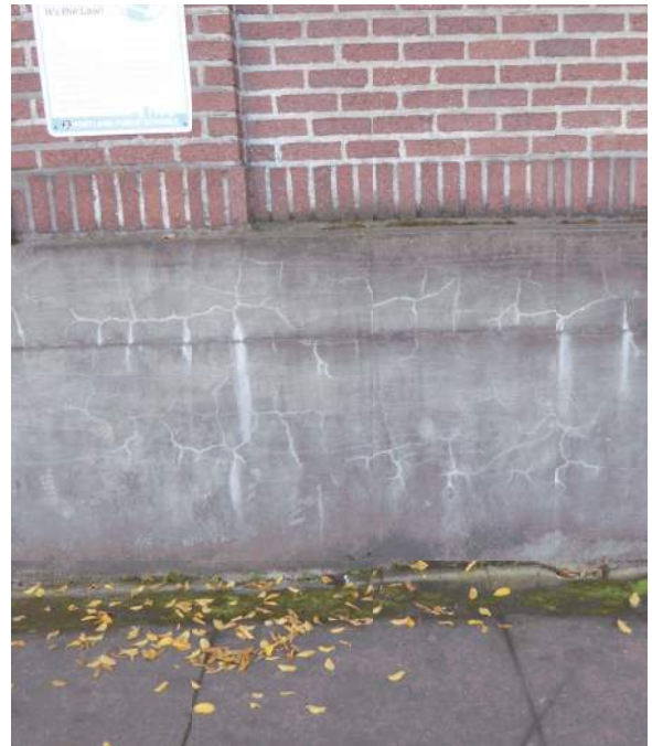
2.2.3/20 Cracks and efflorescence at parge coat.
