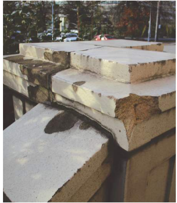
2.2.3/34: Large losses at terra cotta balustrade pier, Building B - west elevation.
