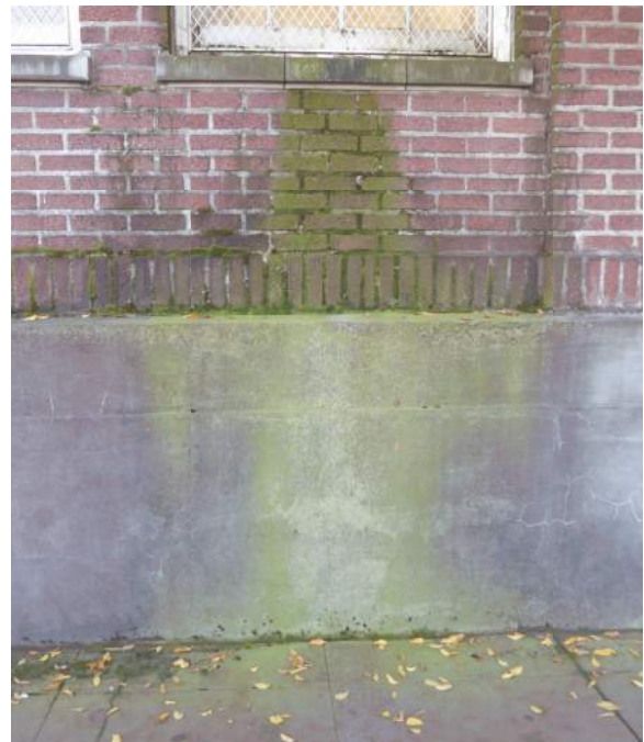
2.2.3/2 Heavy biogrowth where water is directed down the face of the building from a downspout above.
