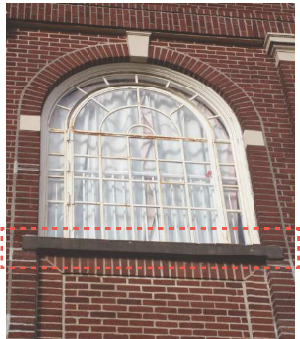
2.2.4/16: Cast concrete window sill at location of removed fire escape stair landing, Building B - south elevation.
