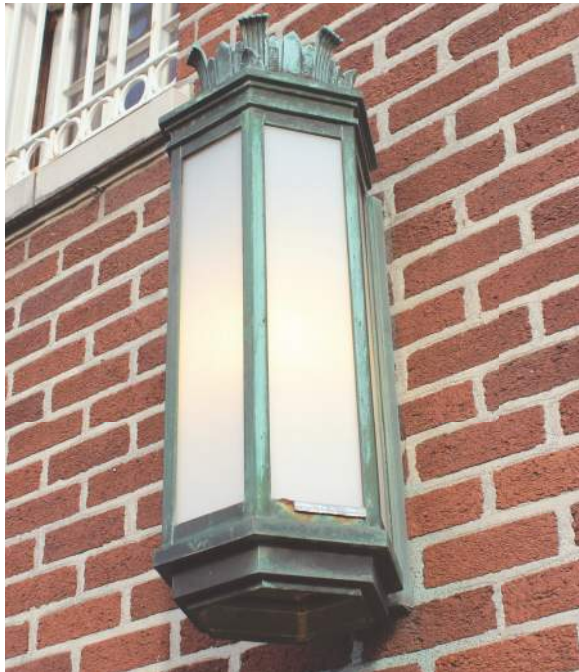
2.7.1/7 Fixture G: exterior copper sconce.
