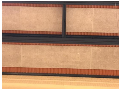
Ceiling Finish (Tectum Acoustical Tile)
