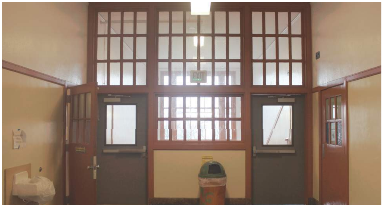
2.5.3/3 Wired glass panes at the staircase historic transom relief windows in Building C.
