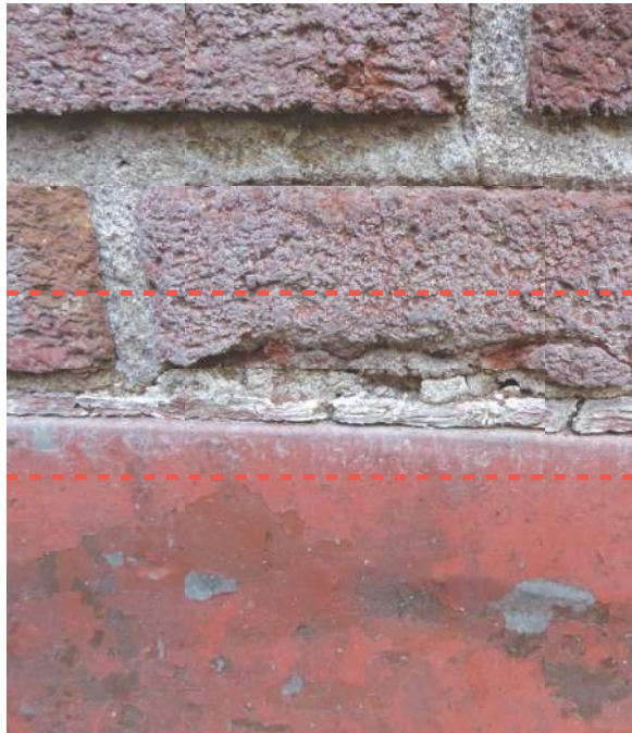
2.2.3/9 Dry/cracked sealant joint.
