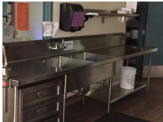
Existing Prep Sink
