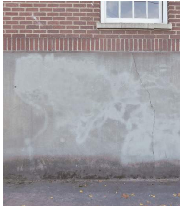
2.2.4/4 Overcleaned graffiti area.
