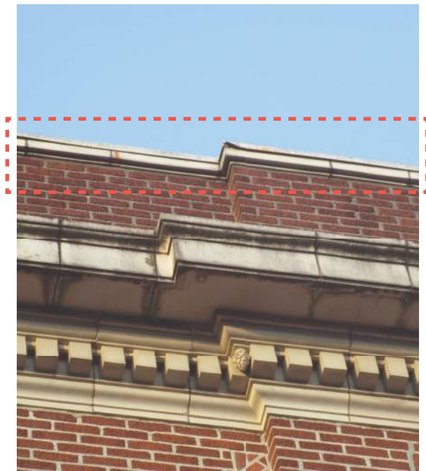
2.2.4/13: Damaged cap flashing at parapet, and rust stains at terra cotta copings, Building B - south elevation.
