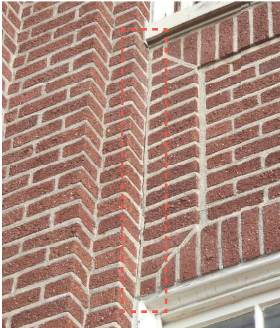
2.2.3/5 Vertical crack at mortar joint.
