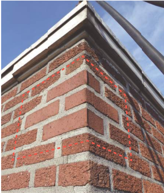
2.2.3/3 Area of brick infill, relatively compatible with existing.
